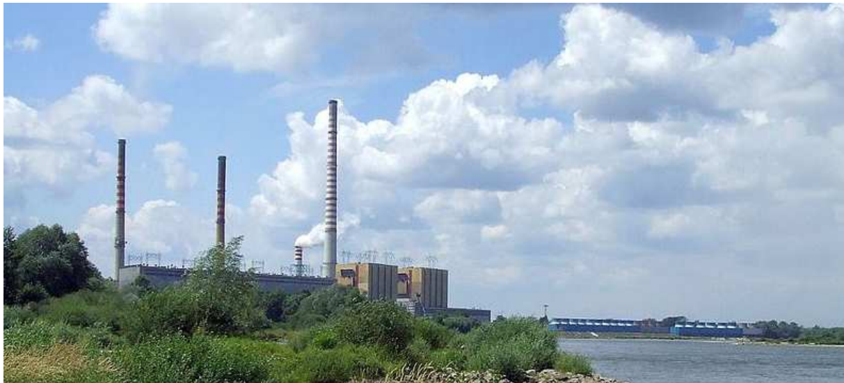
Fig. 4. Kozienice Power Plant
